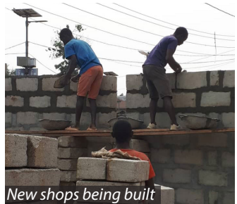
New shops being built
